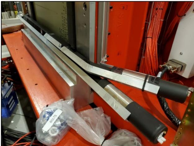
Figure 9: A photo of the mechanical support structure being fabricate and installed to support the hodoscope weight
