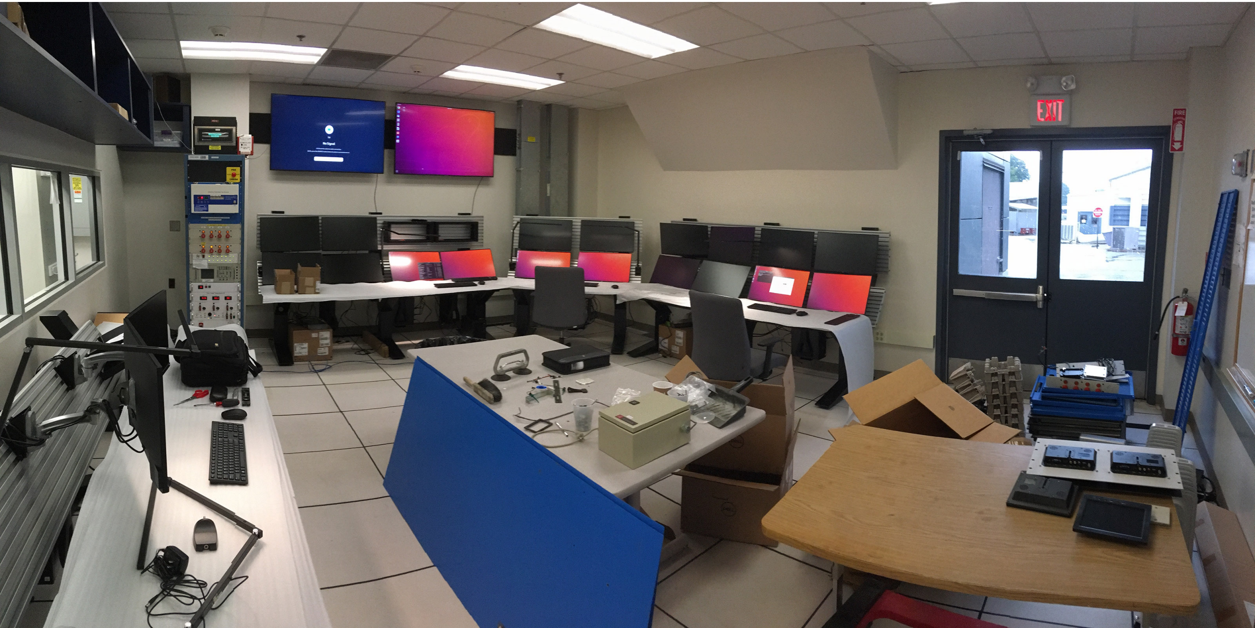
Front room, Aug 22, 2021: All but 2 PCs set up, cabled, not yet networked & configured
