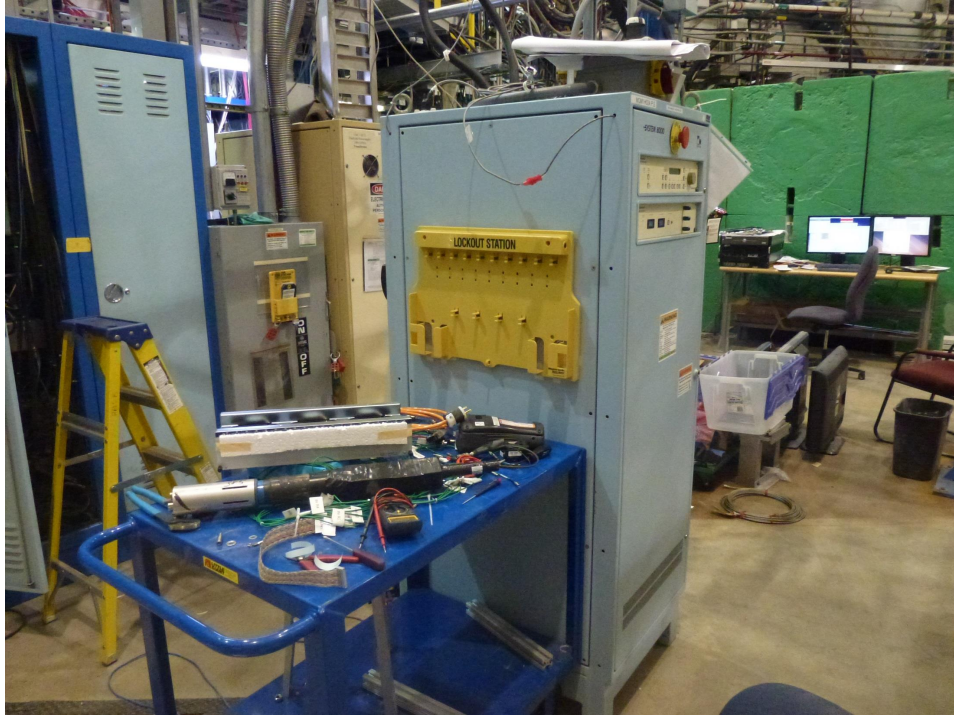
Figure 27: Power supply for the Møller quadrupole magnet MQM1H02A located in the Hall A.
