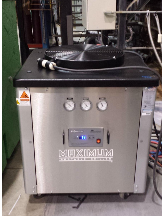
Figure 7: An Advantage Engineering M1-3A water chiller provides the water cooling needed by the CP1110 compressor.
