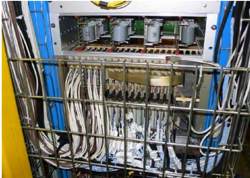
Figure 31: 6U crate in rack L3B03 C-side (L3B13 A-side) with the PS/SPD HV and LED monitoring system. On top of it, the 3U crate with ELBM boards for the VFE PS temperature monitoring system.
