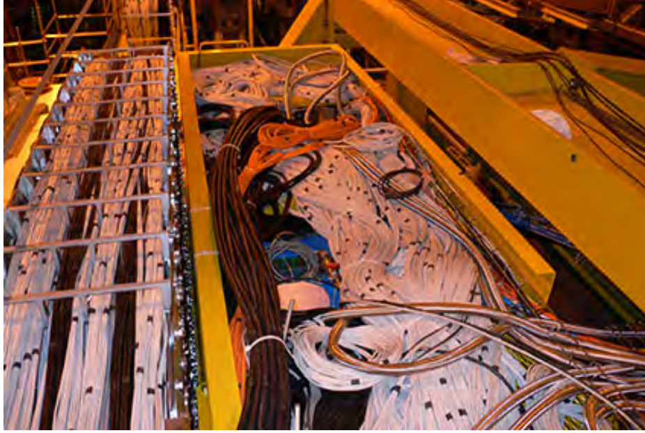
Figure 30: Part of PS cable chain and top roof of ECAL platform C-side with PS/SPD cables on it.
