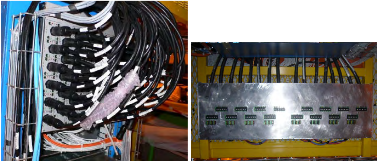
Figure 29: LV cable patch panels for PS VFE in rack L3B03 (left) and for SPD VFE (right).
