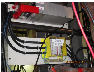
Figure 14.7: Power supply arrangement for MAD cards in the detector hut
