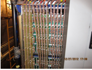
Figure 14.8: Level translator arrangement in the detector hut
