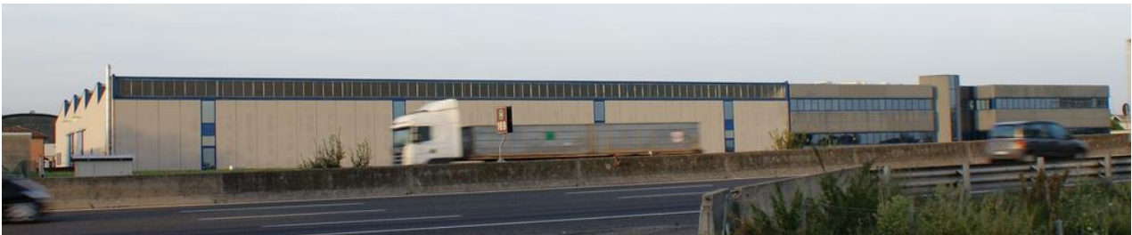
Figure 28: OCEM premises, side view
