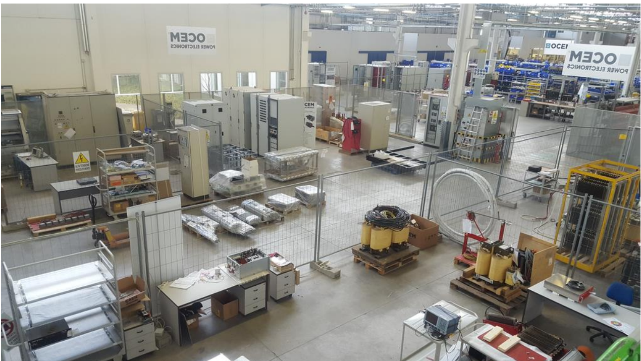
Figure 33: OCEM Test area
