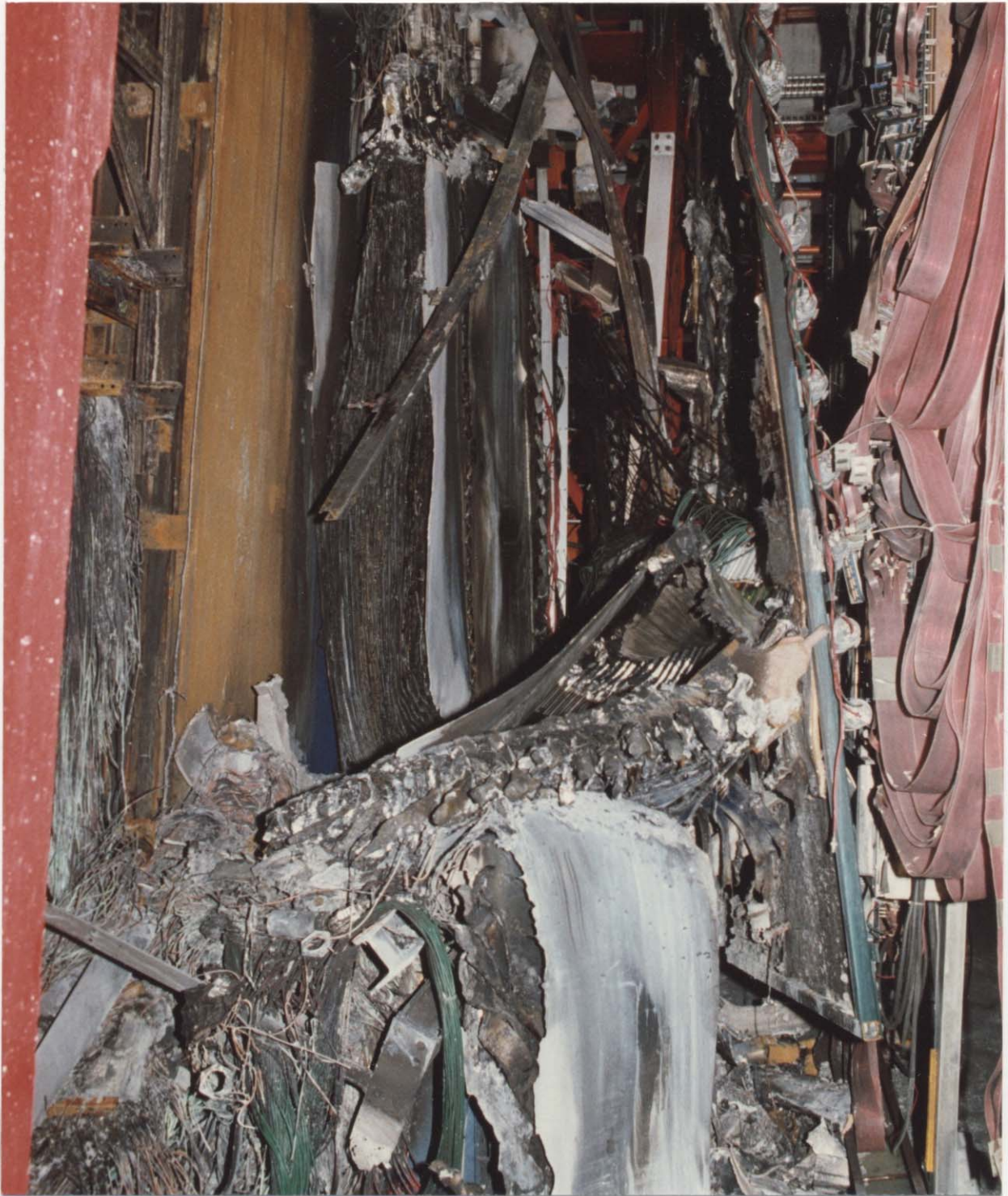
Figure 10. Damage to IEC and HxV. IEC third module and downstream tiebreaker are visible hanging from aluminum framework.
