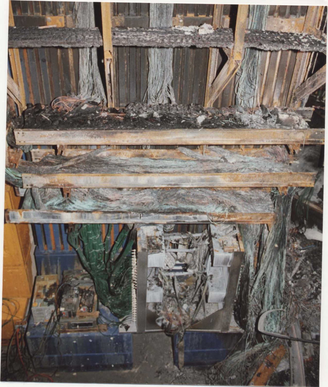
Figure 21. Fire damage to west side of HC.
