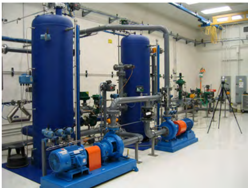
Figure 2.2 Performance Test Loop
