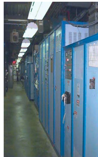
Typical relay rack
